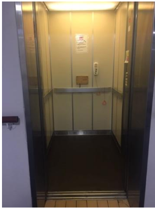
Small but adequate lift
